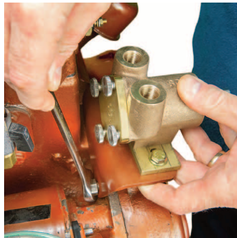
Mount seawater pump/bracket assembly using the upper starter bolt (photo 2)
