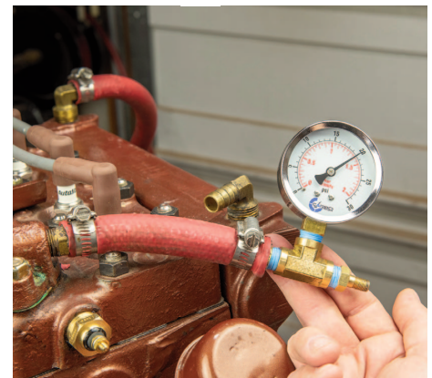
Hand pump removed, block/head holding pressure after pumping.
