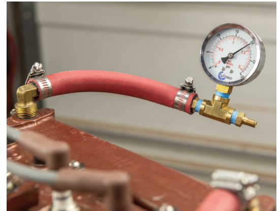
Hand pump removed, manifold holding pressure after pumping.
