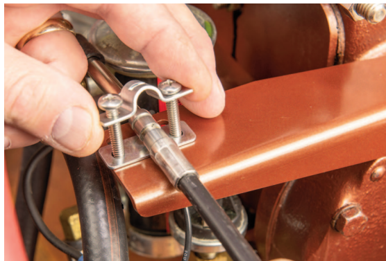
Detail of cable placed over shim plate lining up clamp and bolts with rear mounting holes.
