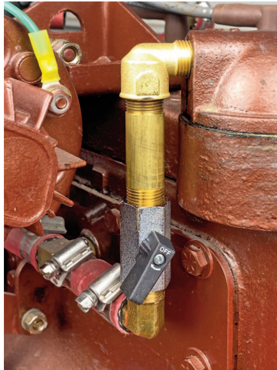
Kit fully installed
