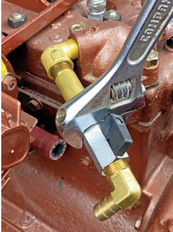
Tighten preassembled fittings into street el
